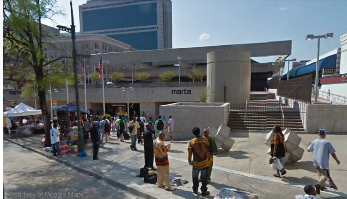
MARTA's Main Transfer Station, Five Points, connects North/South to East/West rail lines.
